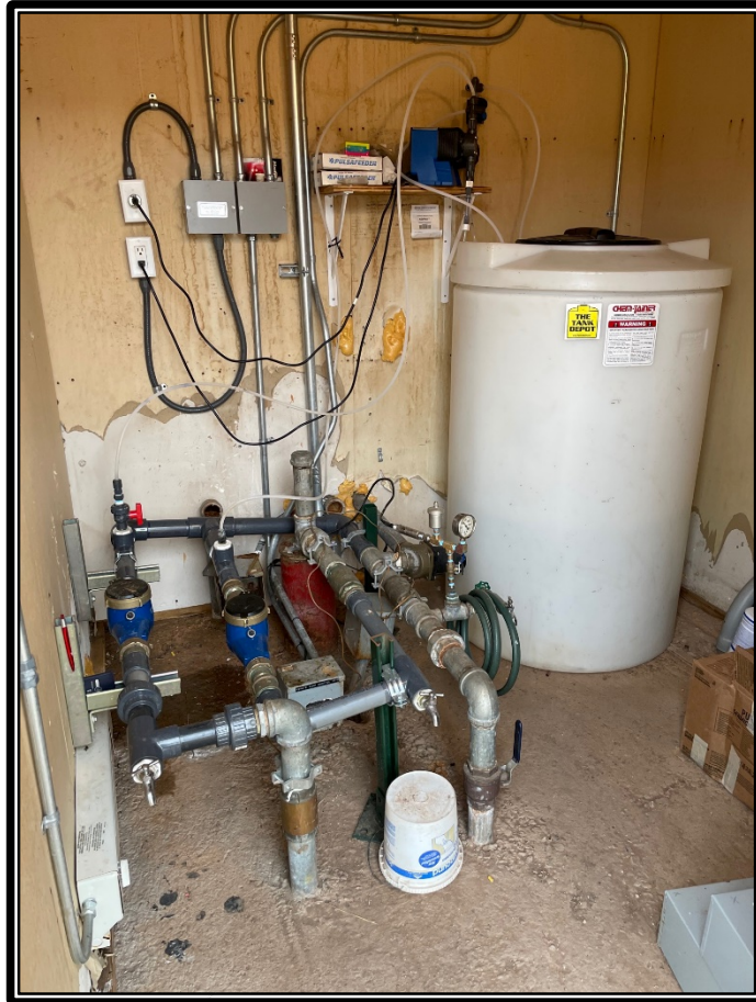
View of Well 1R, Meters and 2" Pipe Manifolds in Pump House 1
