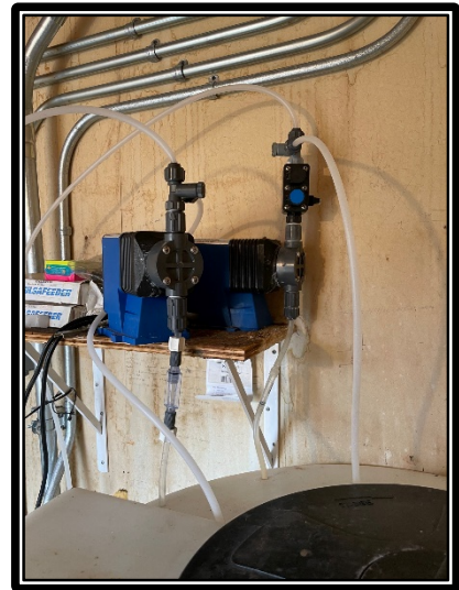
Sodium Hypochlorite Injection Pumps
